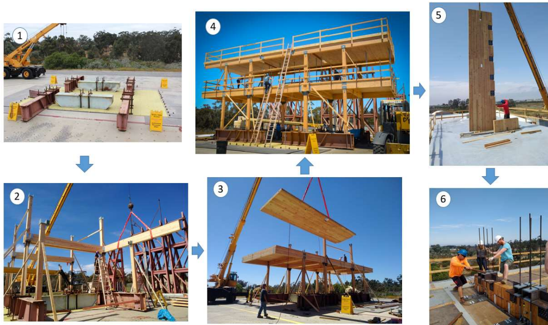
Figure 3. Construction process (1) Foundation preparation (2) Glulam framing (3) CLT panel installation (4) Gravity system completed (5) CLT rocking wall installation (6) Post-tensioning.
