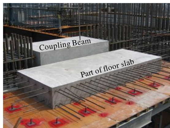
Figure 19 Precast ECC coupling beam dropped into location during building construction (Kanda et al., 2011)
