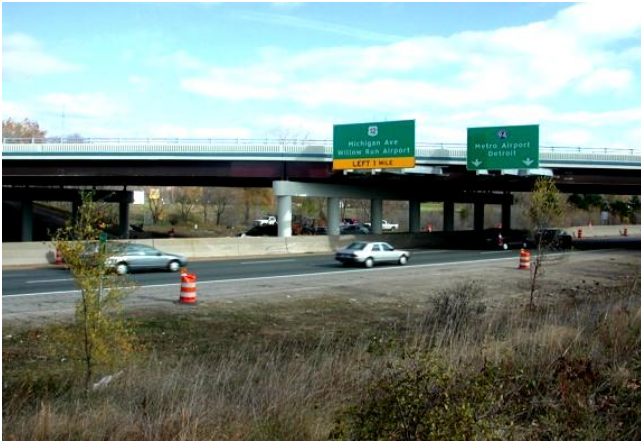
Figure 14 Application of ECC on deck retrofit of a highway bridge in Southeast Michigan
