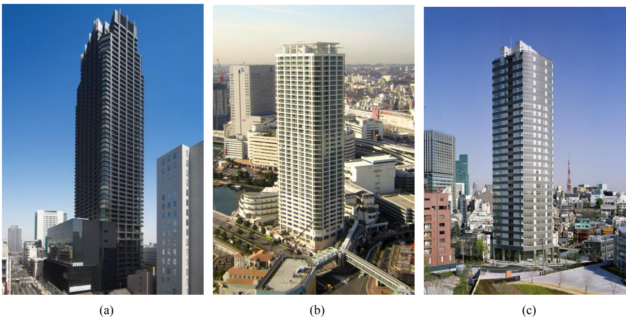
Figure 18 (a) The Glorio-tower Roppongi, (b) the Nabule-Yokohma tower and residence, and (c) the Kitahama Tower in Osaka are recent tall buildings using ECC coupling beams for structural resiliency (Kanda et al., 2011 and Yamamoto, 2008)
