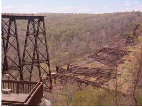
Fig. 1. Kinzua bridge destroyed by an F1 tornado in 2013 (Photo courtesy to UncoveringPA)
