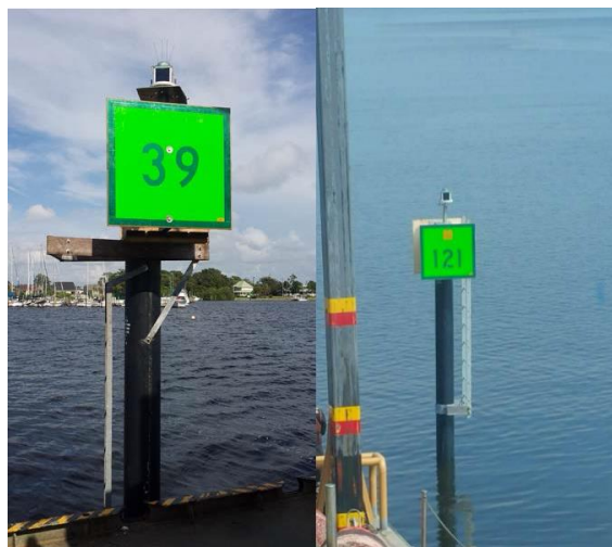
Figure 3. USCG Aids to Navigation (ATON) built using FRP piles [6].
