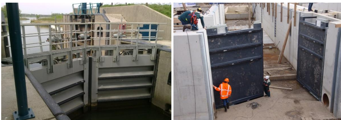
Figure 4. Werkendam FRP lock doors (left) and Erica Ter Apel lock doors (right) [7].
