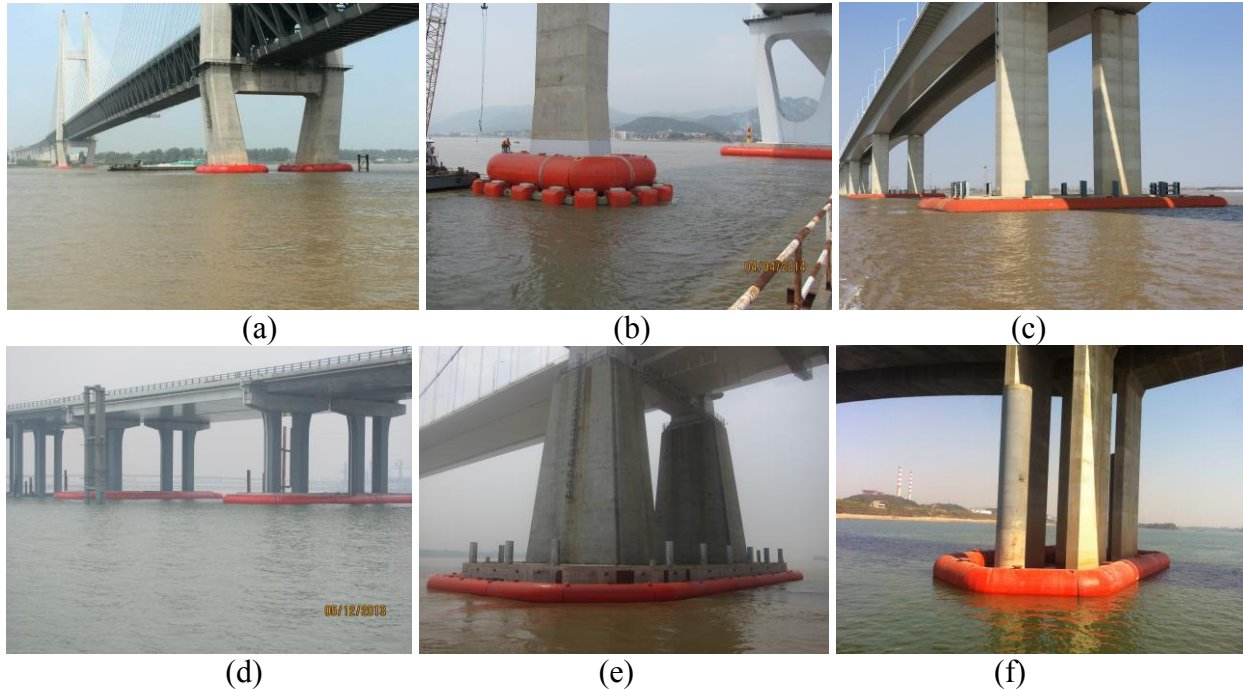
Figure 6. Some applications of LCBS on bridge protection projects in China.
