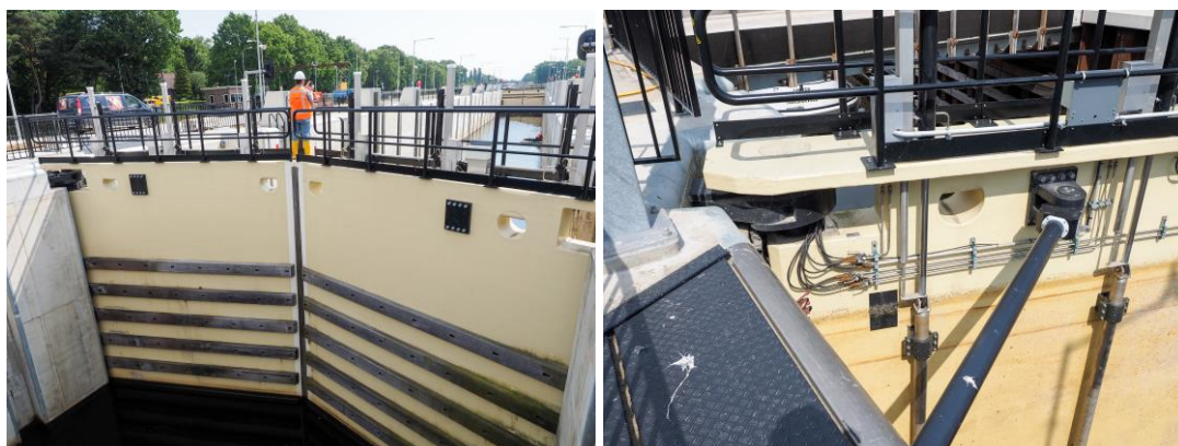
Figure 5. 2014 built world's largest FRP lock doors in the Wilhelminakanaal (courtesy of Wouter Claassen)
