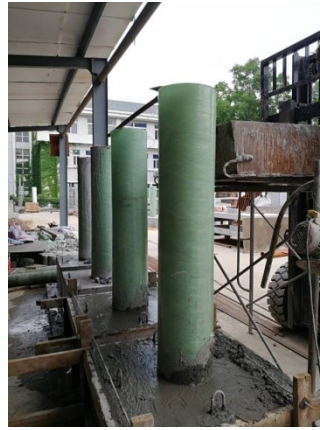
(b) Concrete placement
