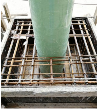
(a) Assembling reinforcement of abutments
