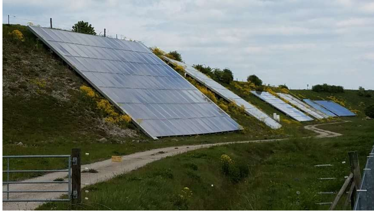
Figure 8: In the German town of Crailsheim, 7,300 m 2 of solar thermal flat plate collectors provide 50 % of the heat for 260 homes. Heat energy is captured and stored seasonally in a 37,500 m 3 underground thermal borehole system.
