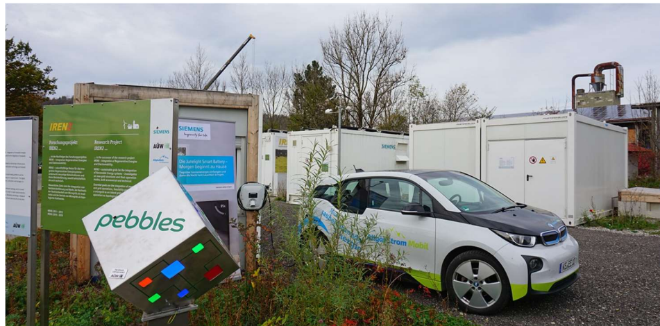
Figure 11. Lithium-ion battery units and community electric vehicles are managed as part of the PEBBLES peer-to-peer energy trading system in Wildpoldsried, Germany
