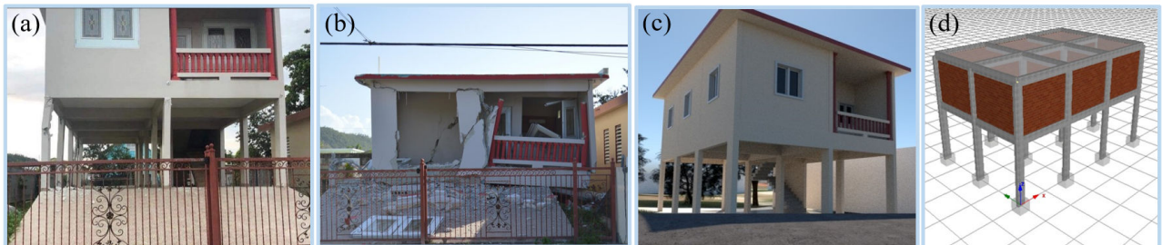
Figure 2. (a) Damaged house after M5.8 earthquake, (b) collapsed house after M6.4 earthquake, (c) 3D CAD model by the students, (d) fiber-based numerical model in SeismoStruct.
