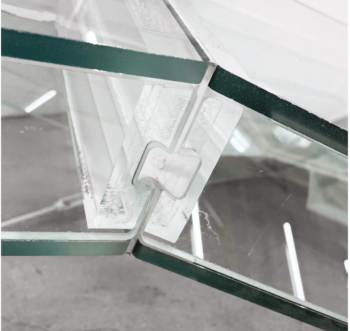
4 Close-up of the butterfly connection mechanism
