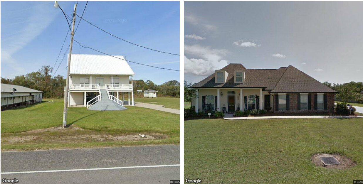
Figure 1. Two examples of homes with a manual label of one-story but predicted labels of two story, due to (left) an elevated foundation, and (right) the presence of architectural dormers.
