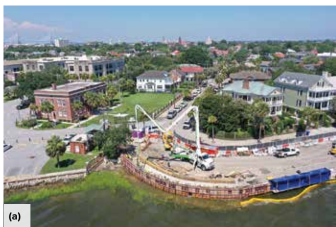
Fig. 2: Phase I of the concrete seawall project: (a) concrete placement of curved section; and (b) completed GFRP seawall curved section
