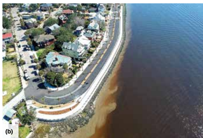
Fig. 2: Phase I of the concrete seawall project: (a) concrete placement of curved section; and (b) completed GFRP seawall curved section
