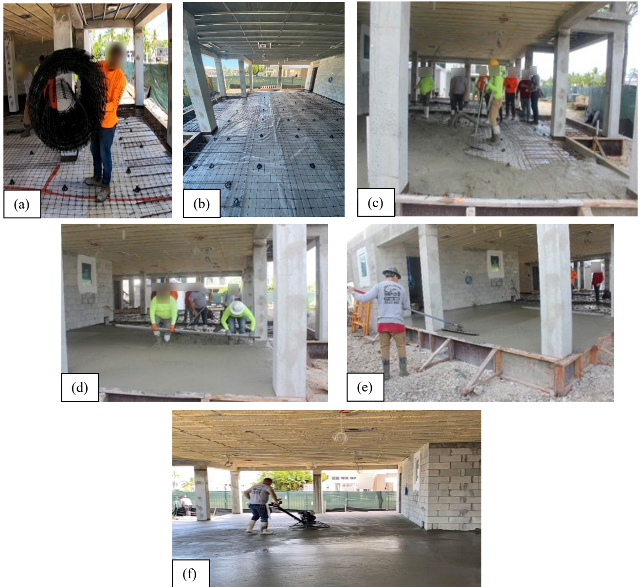
Figure 4 Slab preparation and concrete casting: (a) a crew member lifting a roll of GFRP mesh; (b) mesh implementation; (c) concrete casting; (d) concrete surface screeding; (e) bull-floating of the surface; (f) concrete surface troweling
