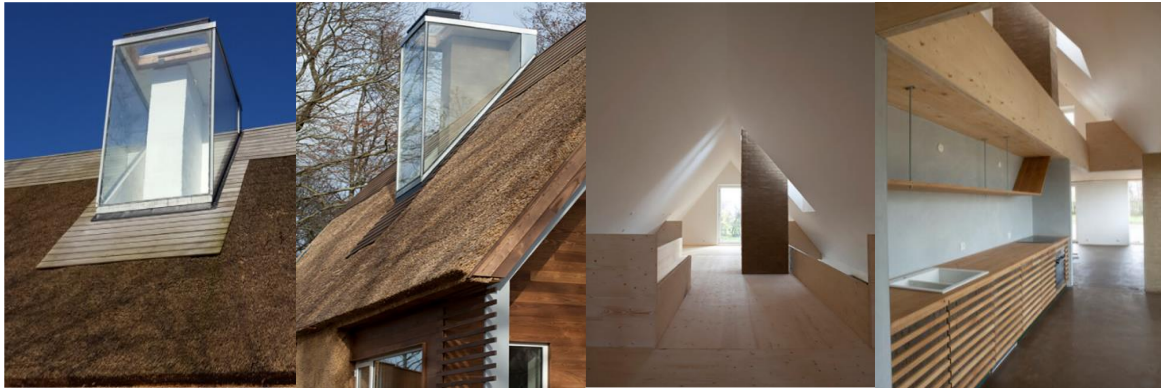
Figure 4. The solar chimney in the Breathable House. Photos by Egen Vinding og Datter/House Arkitekter.
