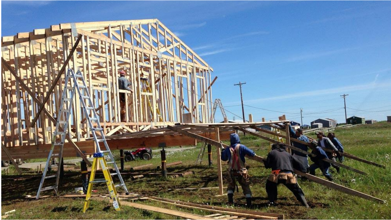
Figure 4. Construction of a home using the integrated truss system. Image courtesy of Cold Climate Housing Research Center, Inc.
