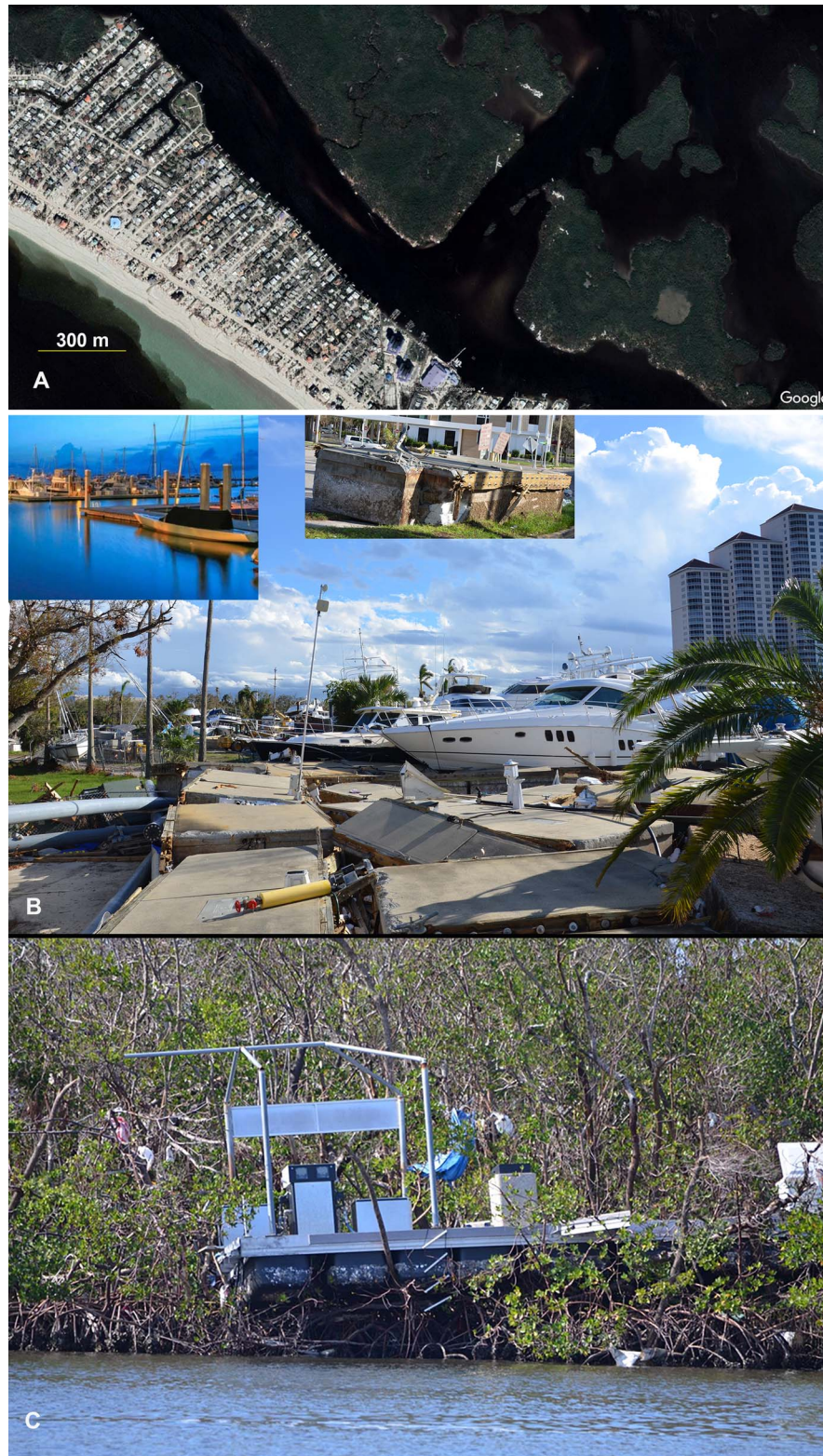
Figure 11. Widespread artificial debris generated by Hurricane Ian. (A) The amount of non-biodegradable and harmful debris washed into the mangrove islands within Charlotte Harbor is closely related to the nearby heavily developed areas; example is from Estero Island (aka Ft. Myers Beach). (B) The high storm surge exceeded height of the anchor pilings of a marina, resulting in all the vessels being washed on land; example is from downtown Ft. Myers. (C) A section of a floating dock and associated fuel station was washed into a mangrove island; example is from southern Estero Bay. See Figure 2 for general locations.
