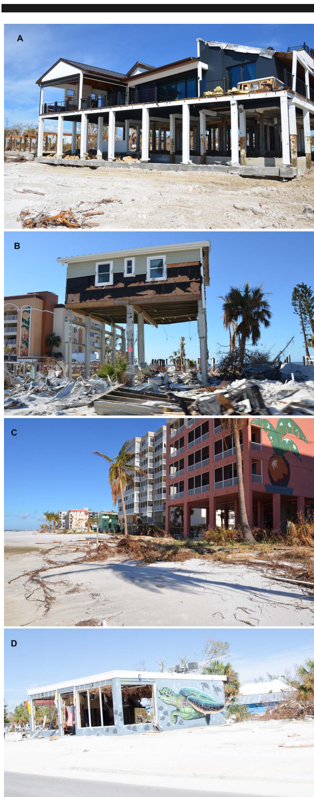
Figure 13. Damage to beachfront buildings. All examples are from the very densely developed Ft. Myers Beach (Figure 2B for location). (A) A relatively new single-family house on concrete pilings. The house to the left on wood piling was washed away. (B) An older single-family house on
