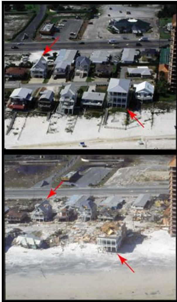
Figure 1.2: Before (top) and after (bottom) Hurricane Ivan hit the coast in September 2004, these homes were in Orange Beach, Alabama, which is on a barrier island.[Source- USGS]
