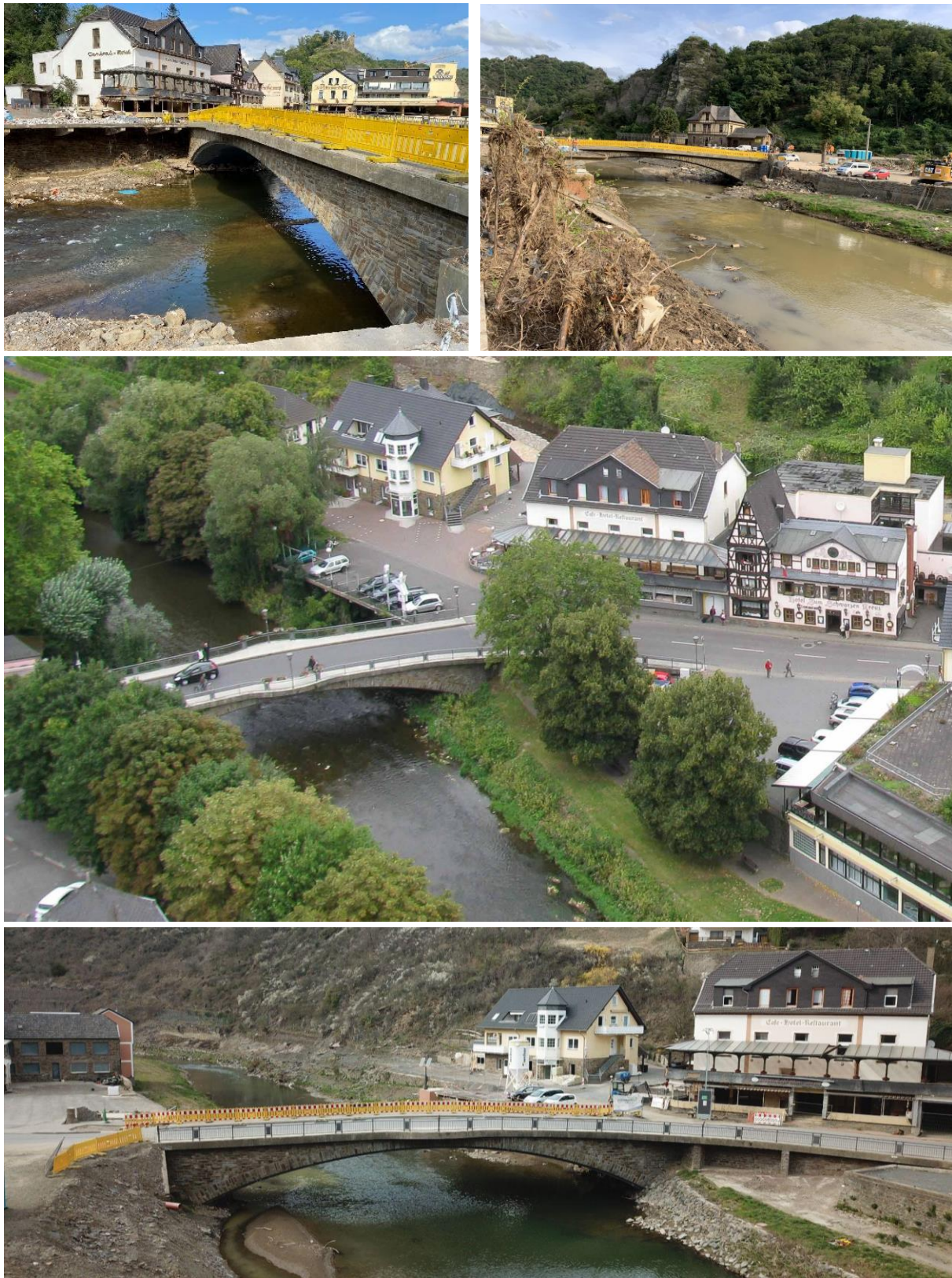
Figure 6. Photographs of the only structurally intact bridge in Altenahr following the flood, Top: Photos of abutment regions of the bridge in Aug 2021, Middle: Pre-flood aerial photograph, Photo Credit: Heinz Grates ( https://www.aw-wiki.de/w/index.php?curid=36263 ), Bottom: Aerial photo taken by the GEER team in March 2022, showing the bridge after clean-up work.
