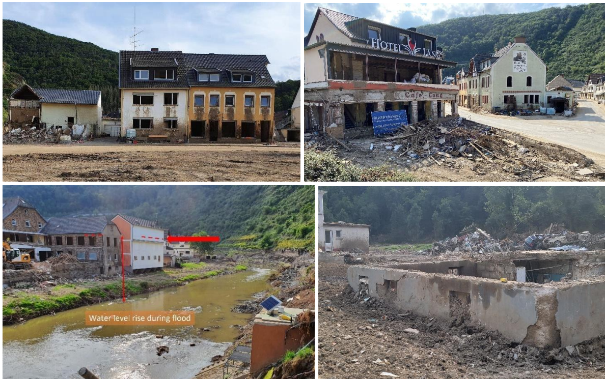
Figure 4. Example of structural/residential damage in Altenahr (town).
