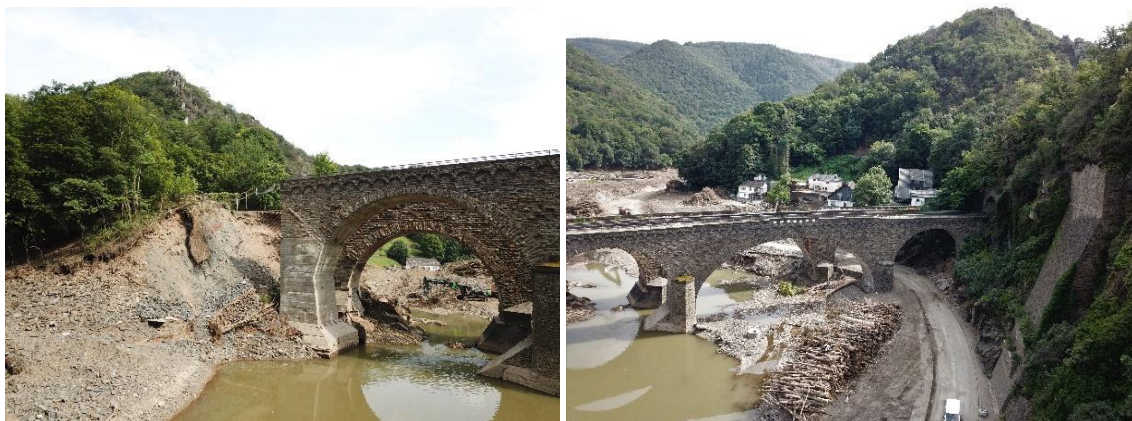
Figure 12: Photo of the abutment region of the double bridge, August 13 th , 2021. Left: Washed out abutment area, Right: bridge abutment area intact and connected to adjacent rock slope
