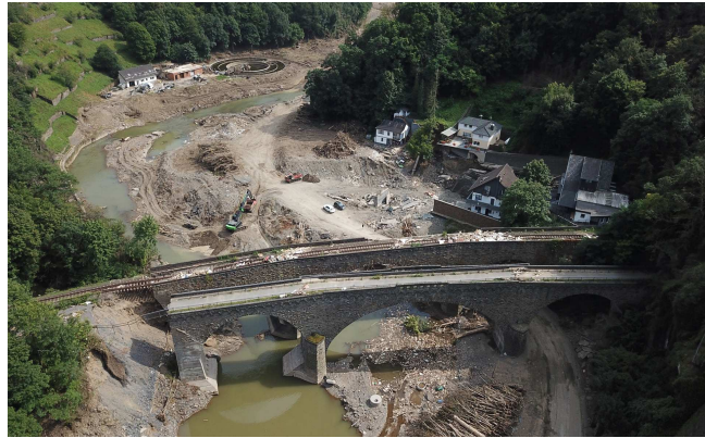
Figure 7. Aerial image of the Altenahr tunnel exit and double bridge, August 13 th , 2021
