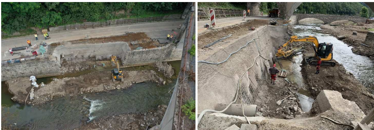
Figure 3. Ongoing repairs of localized embankment failure along highway L73
