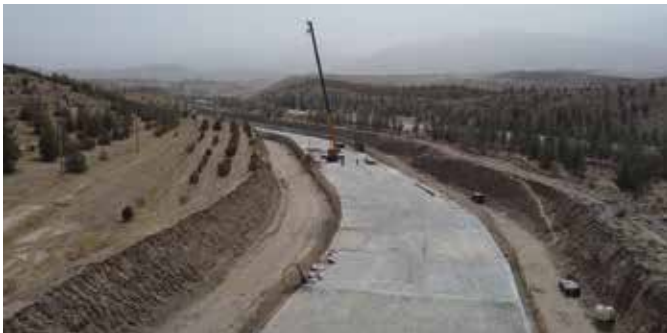
Fig. 6: Channel slab after concrete casting
