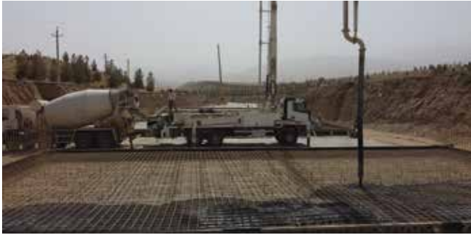
Fig. 5: GFRP reinforcement in channel slabs
