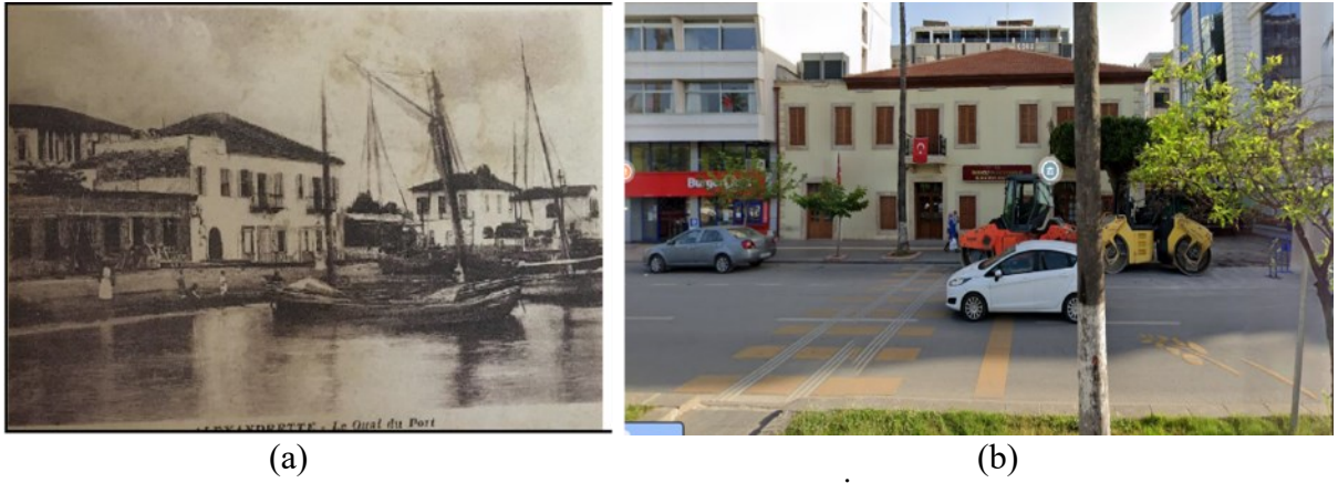
Figure 3. Example of historic development and reclaimed land in İskenderun. Building P, a former community center and current civil registry on Atatürk Boulevard, is shown in both images: (a) image that predates 1916 and along the former shoreline [date not known, obtained from Nalça (2018)], and (b) modern image of the building on Atatürk Boulevard [May 2020, obtained from Google Street View] (approximate coordinates 36.5916N 36.1702E).
