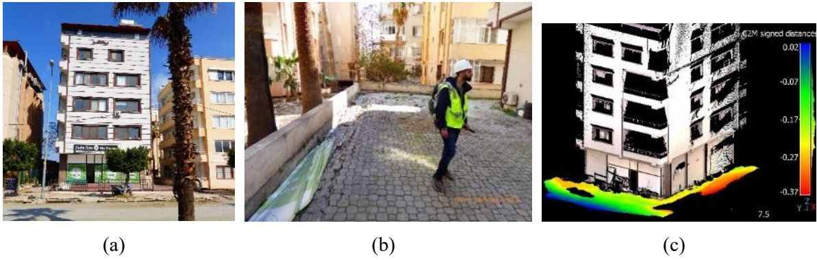
Figure 11. Building F on Bahçeli Sahil Evler Street in the Çay District: (a) street view of the building (36.5900N 36.1782E; 28 MAR 2023), (b) north side of the building showing the ground deformation and settlement (36.5903N 36.1780E; 28 MAR 2023), and (c) lidar scan data showing ground deformation patterns around the structure.
