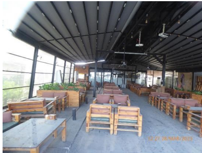
Figure 20. (a) Group of three buildings on Atatürk Boulevard with the restaurant Building L in the middle (36.5909N 36.1777E; 29 MAR 2023), (b) damage to the exterior at Building L associated with hogging ground deformation (36.5906N 36.1778E; 28 MAR 2023), (c) damage to the concrete slab at Building L associated with hogging ground deformation (36.5907N 36.1779E; 28 MAR 2023).
