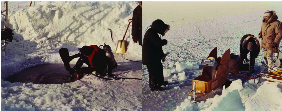
Fig. 11 Historical photos from the Arctic Dynamics Joint Experiment by Tom Marlar (AIDJEX, 2023). Left: Boundary-layer studies involved divers assembling current-meter masts under the water and mapping the under-ice topography. Right: Microwave emissivity measurements over different sea-ice conditions were made to better understand the microwave signature of sea ice.
