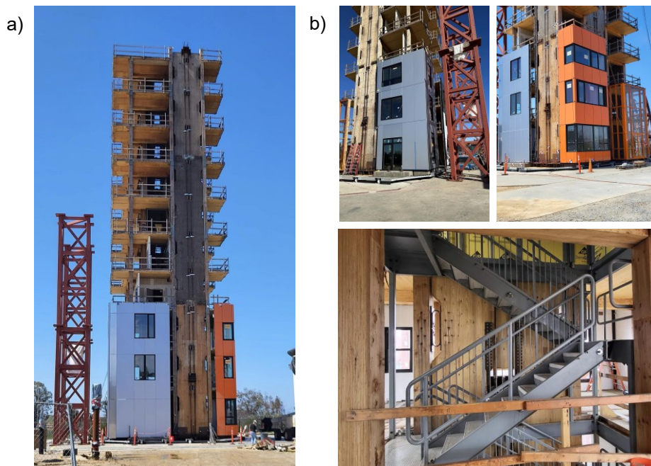
Figure 2. Test building: (a) 10-story mass timber building; (b) nonstructural systems
