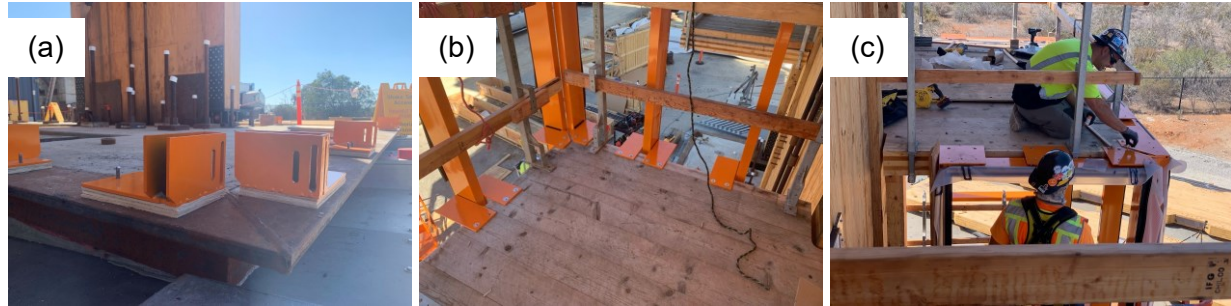
Figure 3: (a) Slotted sill anchor at the foundation, (b) slotted windload anchors at 2 nd floor diaphragm, and (c) slotted head anchors at 3 rd floor diaphragm.
