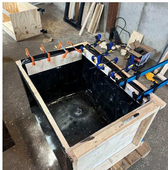
FIGURE 3 Waterproof Application on Box 1 Interior Sides
