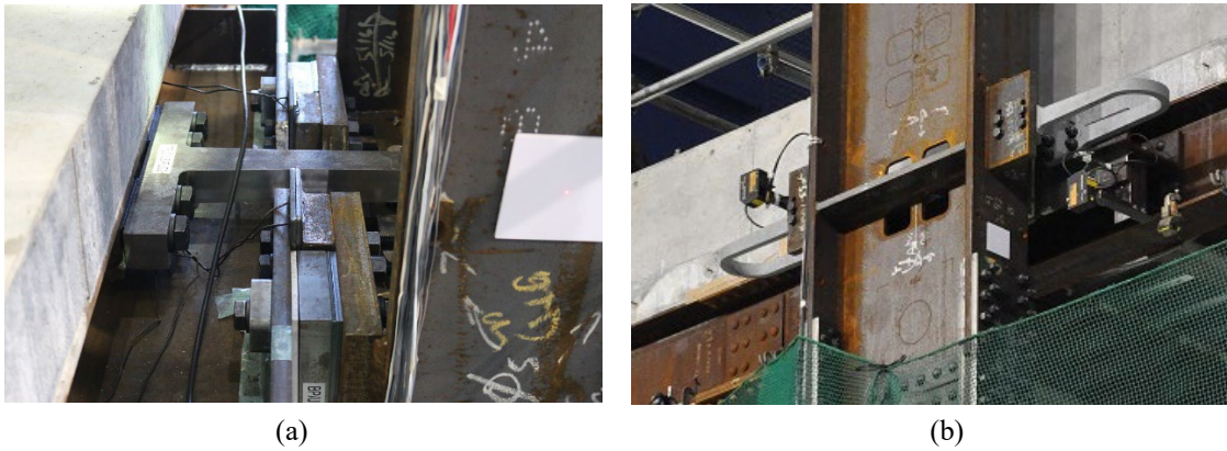
Fig. 3 – Force-limiting connections with yielding elements
