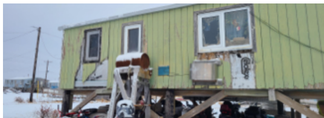
Strengthening our outer walls and wind resilience
