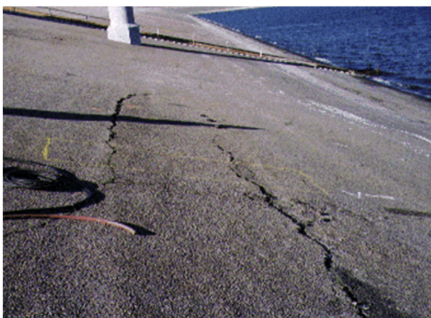
Fig. 1. Large cracks formed on the upstream side concrete of the Los Angeles Dam [9].
