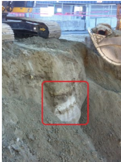
a. St. Paul St. excavation showing soil layer
