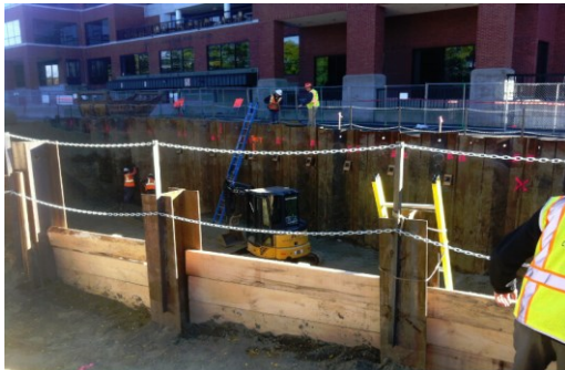
a. Sheet piles with soil nails providing lateral support
