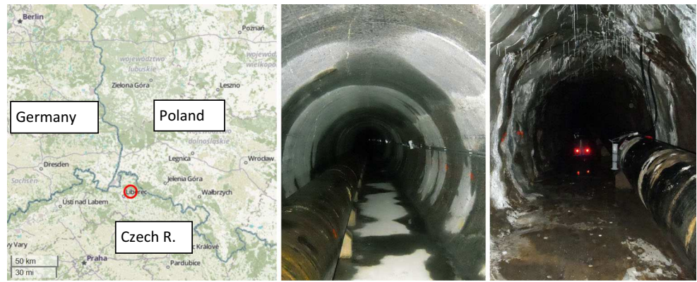
Fig. 1 Position of the studied site on a map (left, source: OpenStreetMap project), photographs inside the tunnel in the bored part with very little inflow on bare rock (middle) and in the blasted part with inflow through a concrete-covered fault intersection (right, photograph by P. Rálek). The tunnel is 3.6 m diameter, and the pipe is 0.8 m diameter
