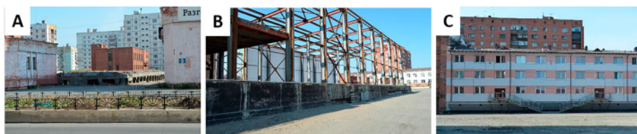
Figure 3. Foundation recycling in Norilsk. (a) Example of pile foundation left after removal of damaged concrete/brick building. (b) Construction of light frame and composite panel structure on old pile foundation. (c) One of the three light residential buildings erected on recycled foundations in 2013 (Photographs by N.I. Shiklomanov).
