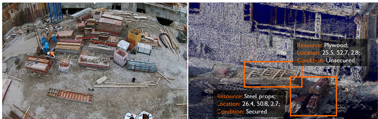
Figure 3. A job site from aerial perspective (Left), potential at-risk construction resources localized in a ground and aerial 3D model (Right).
