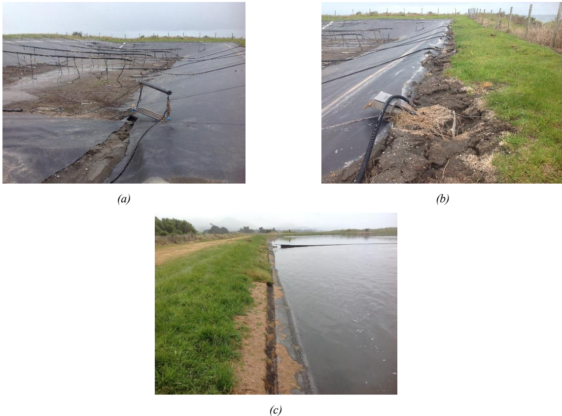
Figure 44: (a) KK-OPS looking from the SW corner. Note: Geoliner in the foreground has ripped ( -42.3668^\circ , 173.6865^\circ , taken facing E). (b) Rotation of the aeration-line control posts on the south side of KK-OPS ( -42.3669^\circ , 173.6867^\circ , taken facing E). (c) West edge of KK-OPN. Note concrete panel has displaced into pond ( -42.3660^\circ , 173.6868^\circ , taken facing N).
