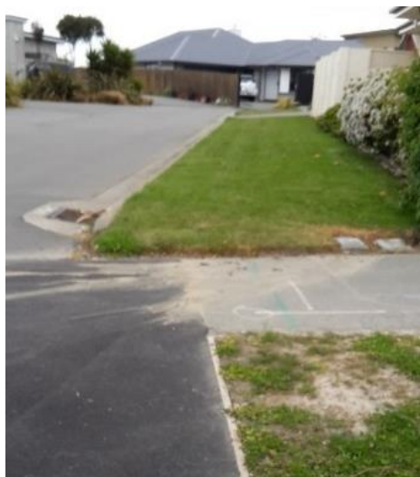
Figure 54: Isolated ejecta in the Parklands area of Christchurch (Approx. coord: -43.47°, 172.71°; Photo courtesy of S. Cox).
