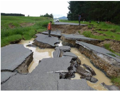
Figure 47: Damage to Leslie Hills road caused by fault rupture (Approx. coord: -42.631^\circ , 172.990^\circ , taken facing W).
