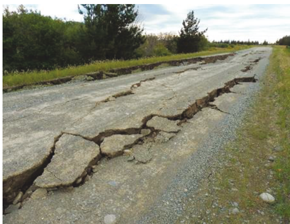
Figure 15: Lateral spreading induced cracking along top of northern stopbank ( -41.4387^{\circ} , 174.0214^{\circ} , taken facing E).
