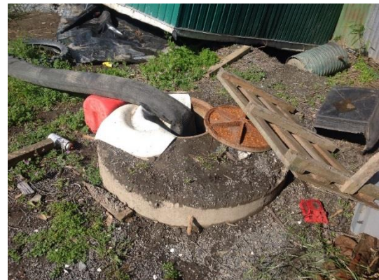
Figure 33: Floatation of manhole on Beach Road near to Lyell Creek (-42.3848°, 173.6783° taken facing SW).
