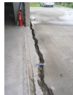
Figure 25: Separation of concrete slab from clubhouse ( -41.4768^{\circ} , 173.9855^{\circ} , taken facing N).
