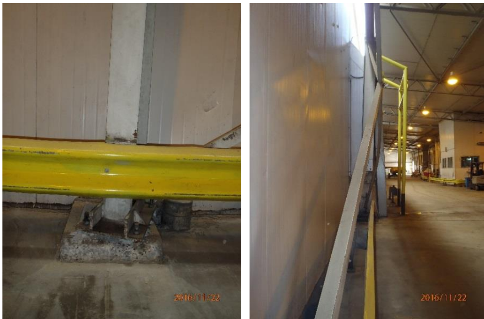
Figure 32: Internal east wall in northern part of the Shed, which shows column-pedestal connection failure due to rotation of the base of the column and buckling of concentric bracing. (Approx. at S41.280939° E174.784778°, 22NOV16).
