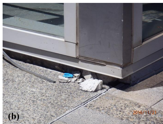
Figure 36: Ground settlement relative to the pile-supported B building at: (a) the southwest corner of the building with ground improvement (S41.279767° E174.782100°, 21NOV16), and (b) northwest corner of the building without ground improvement (S41.279419° E174.781443°, 21NOV16).
