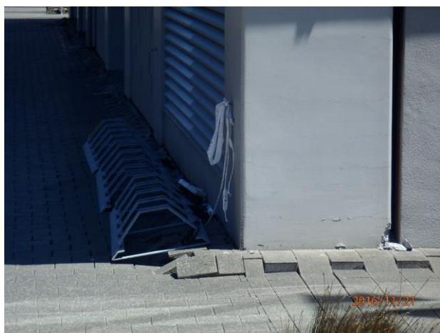
Figure 35: Looking west at southeast corner of the S building at which fill settled approximately 100 to 200 mm relative to pile-supported building. (S41.278285° E174.784757°, 21NOV16).
