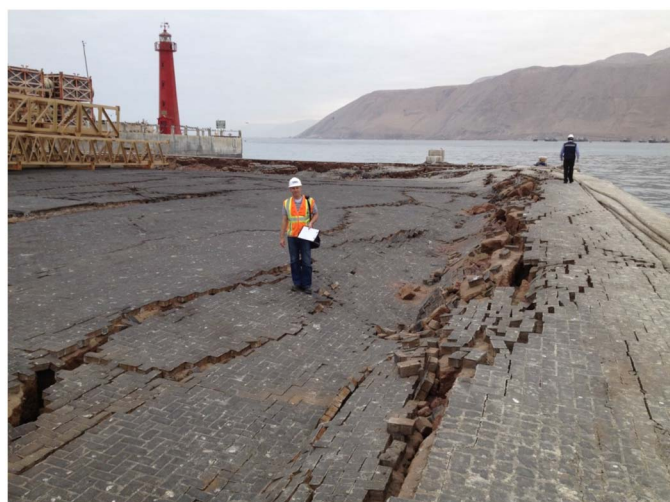
Fig. 2. Liquefaction and lateral spread damage near the head of the Molo Pier in Iquique, Chile (reprinted from Rollins et al. 2014, with permission)
