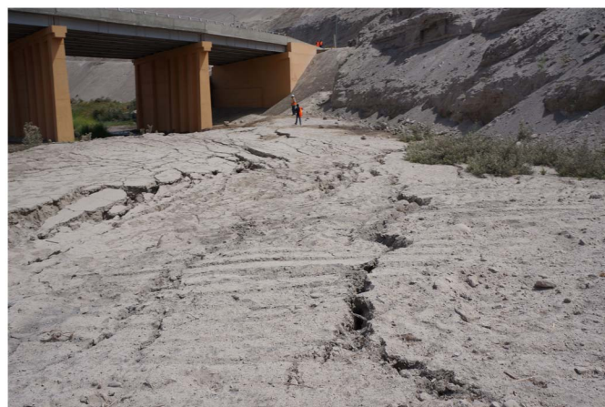
Fig. 3. Liquefaction and lateral spread displacement at the Tana Bridge on Interstate-5 in Chile (image by K. Franke)
