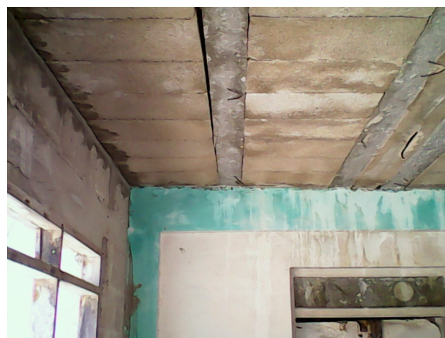
Figure 5. Interior of house showing moisture damage (Photo: J. Biles).
