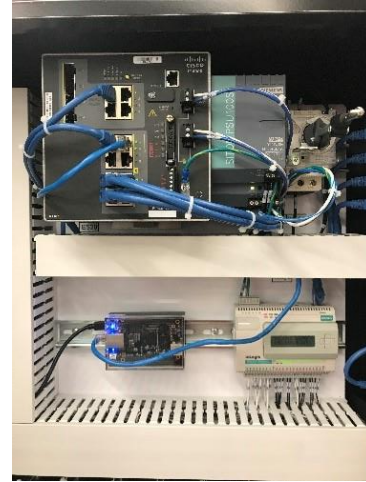
b. BBB (Bottom Left) and IE4000 (Top) Mounted in SmartBox Cabinet
