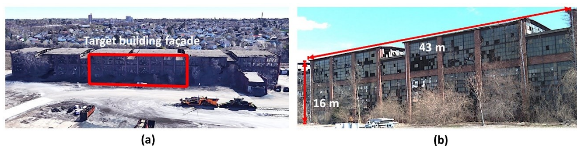
Figure 4. Experimental validation using a building having severe façade damage: (a) 3D view of the building (courtesy of Google 3D Maps) [32] and (b) Façade test region.
