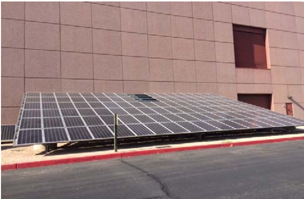
Figure 1. The SenSIP 18kw (104 panel) experimental facility established at ASU with industry collaborators [1].
