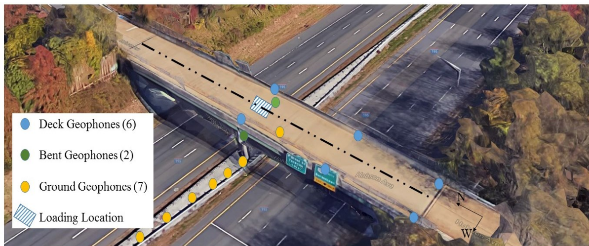
Figure 4: Geophone placement layout.
