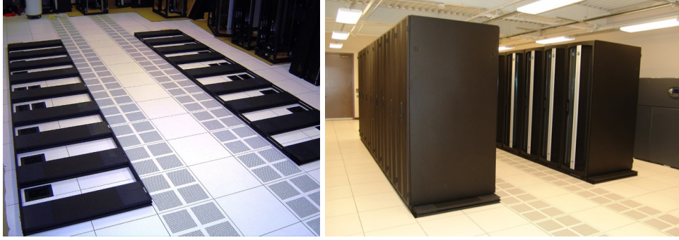
Figure 1: Multi-unit rolling isolation system array installation at a financial institution data center. Source: [23].
