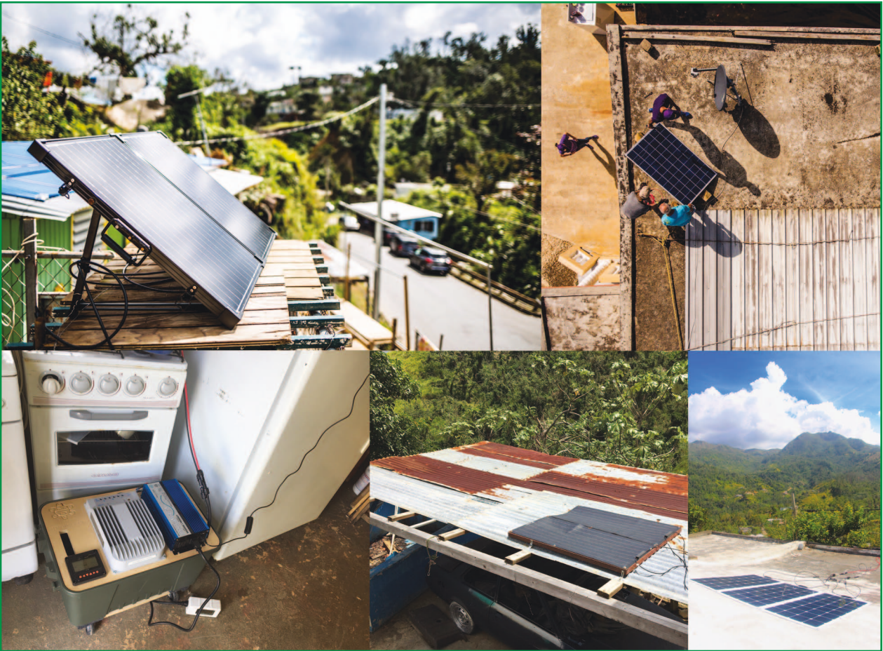
figure 3. Some of the PV-battery systems installed in Puerto Rico by researchers at the University of Washington in Seattle. (Photos courtesy of the University of Washington, used with permission.)
