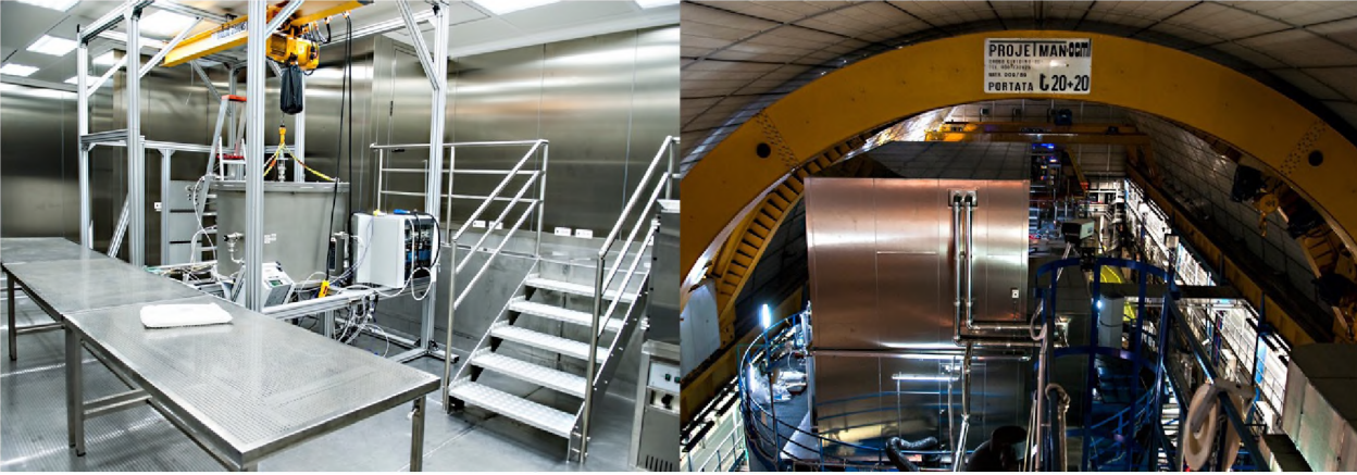
Fig. 85. The DarkSide-50 radon suppressed clean-rooms in Hall C . Left: The interior of the CR1 clean room, with the UHV evaporator for TPB coating of detectors' internals visible at left of center. Right: The exterior of the assembly clean room CRH on the top of the CTF water tank, housing DarkSide-50.
