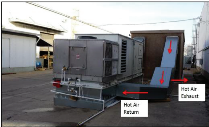
Figure 2: Rear view of MDC shows hot air return duct
