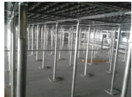
Figure 11. (a) Map view of ES2 DC lab. Racks and tiles matrix. (b) ES2 DC under-floor plenum.
