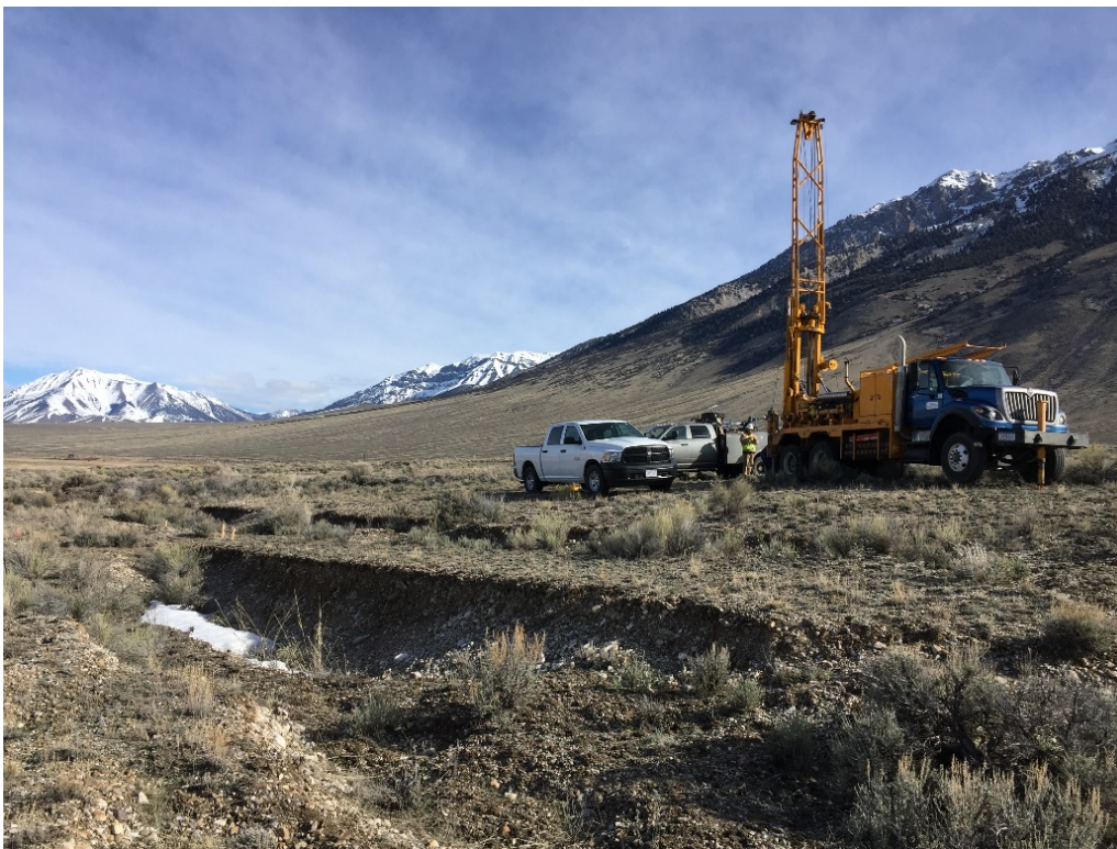
Figure 4. Photograph showing large fissures produced by liquefaction-induced lateral spread displacement towards the Thousand Springs Creek to the left.
