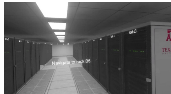
Figure 6: Inspecting the data center. The rows of racks are lettered, and the positions within the rows are numbered. The user is instructed to navigate to rack B5.
