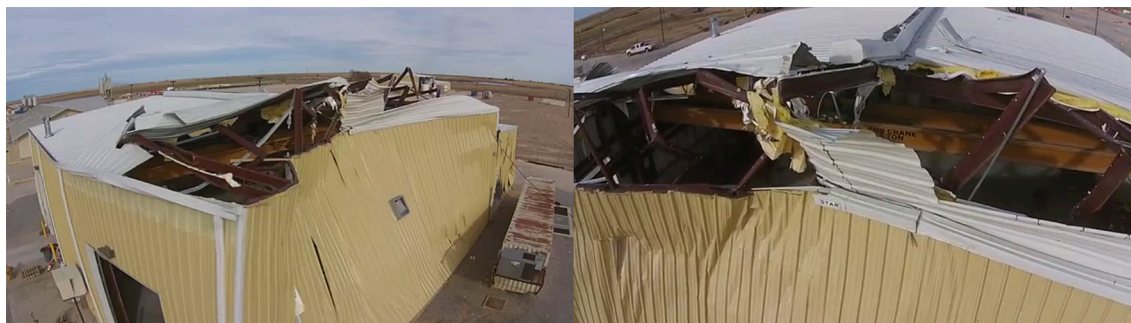
FIGURE 11 | UAS-based imagery of metal building structures damaged by the EF-3 tornado at the Halliburton Oilfield Services facility outside Pampa, TX, in November 2015. (Image Credit: R. L. Wood).
