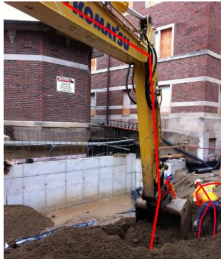
Figure 1. Illustration of the 2D on-site pose estimation system on a video frame for both articulated equipment and human workers. Red lines are the estimated pose.
