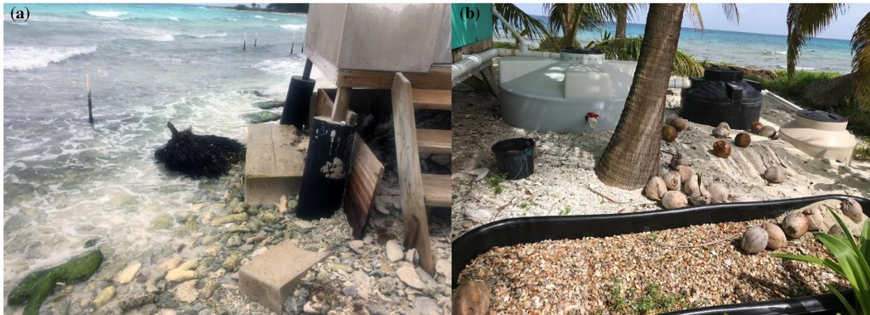
**Figure 3.** Restroom facilities and OWT installed by Ecofriendly Solutions Ltd. at Laughing Bird Caye National Park, Belize. Pictures taken in a) March 2017 showing algae covered rocks and interventions to combat erosion and b) March 2018 showing relocation of OWT with increased treatment capacity.
