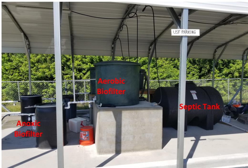
**Figure 2.** Pilot HABiTS at North West Water Reclamation Facility
