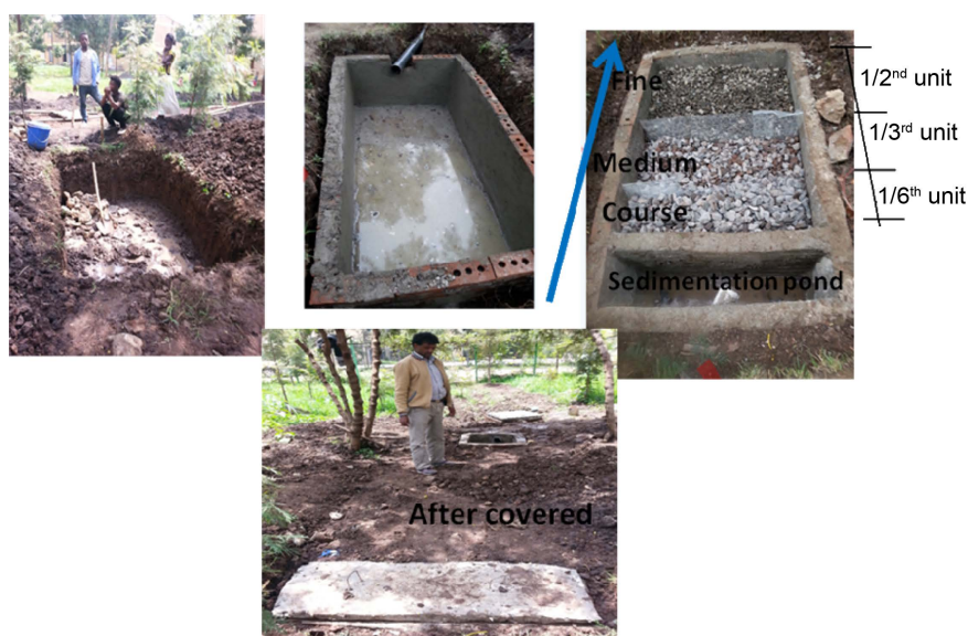
Figure 4. The low-cost stormwater filtration system from excavation to filling the system with filtration media (top) to making the system ready for performance test (bottom).
