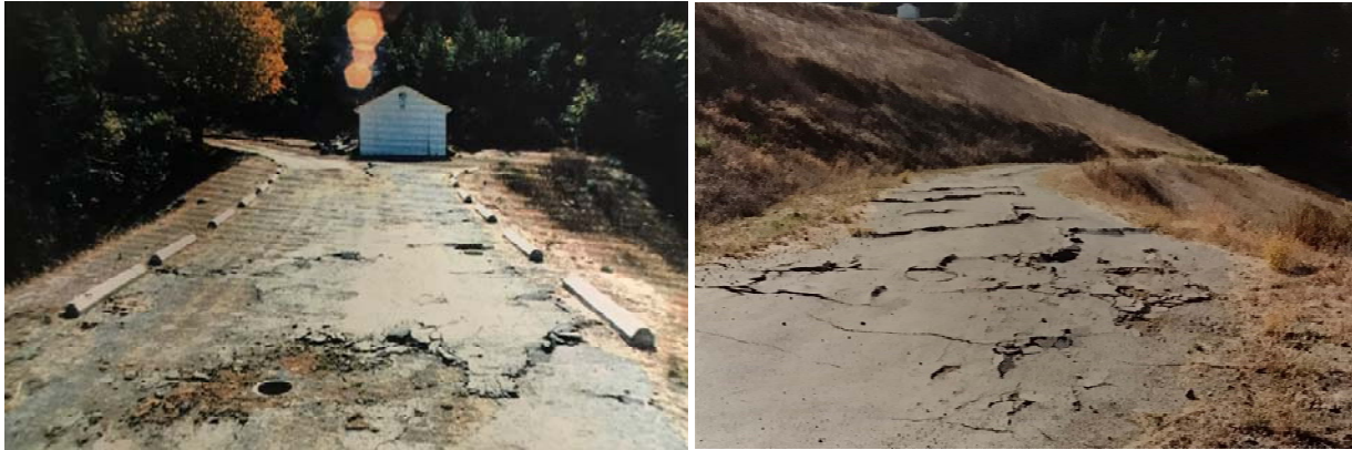
Figure 5. Photographs of cracking after Loma Prieta earthquake: (a) longitudinal and transverse cracking on the dam crest near the left abutment, (b) cracking along access road on the lower portion of the downstream face (California Division of Safety of Dams files 1989)
